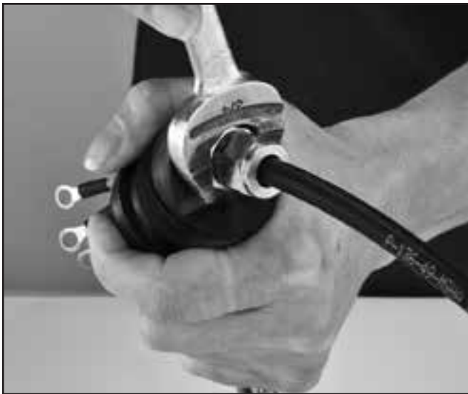
Tightening the Mount Nut.
